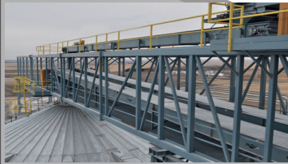
Box Bridge with Conveyors on the Inside and on Top
