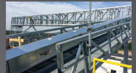
Fill Conveyor Trusses and intermediate Access Trusses
